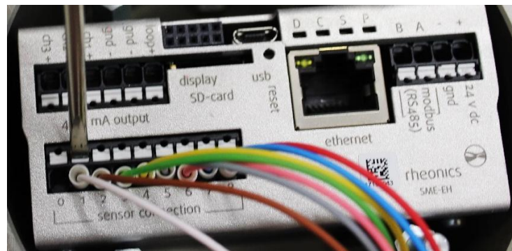
Figure 7: Disconnecting a wire from SME.
