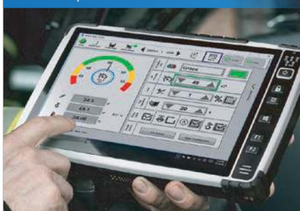
Plant supervisor's dashboard
